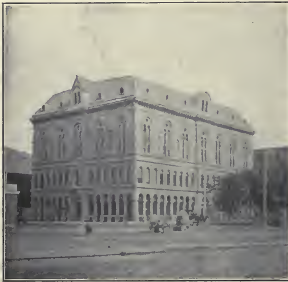
St. Patrick's Hall, which formerly occupied the south-east corner of Craig Street and Victoria Square. It was the centre of many sides of the city's life in its day. The building collapsed one night following an evening of festivities within its walls, thus narrowly averting a tragedy.
